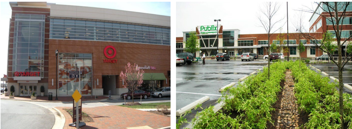
Figure 5.7.F(1): Examples of Large Retail Establishments
