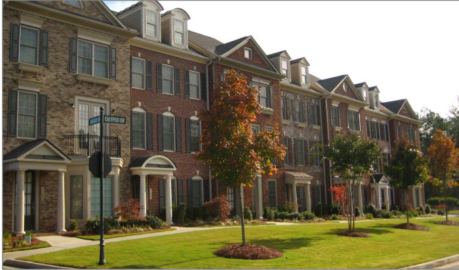
Figure 5.7.D(5)a: Changes in Building Façade
