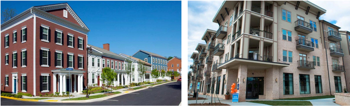
Figure 5.7.D(5)c: Examples of Front Façades
